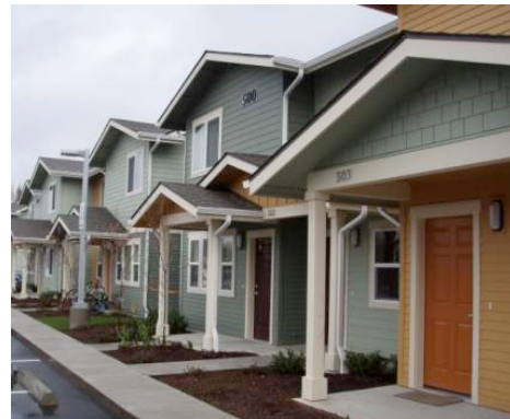
Villa Santa Maria, Catholic Housing Services
